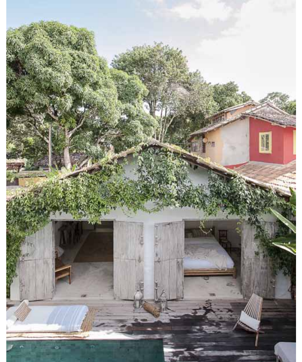
Exterior Jan Eleni Lemonedes, Ronnie Stam and their daughter Lola (pictured opposite) wanted their Brazilian holiday home to reflect the traditional local style of house building, but with a light and airy feel. A careful mix of white-washed concrete, expanses of glass and wood specially washed to make it paler contributes to the resultant modern-rustic look
